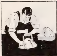
3. Tamp Soil Around Edge of Setter.
